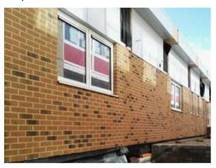
The only site works required in respect of completing the exterior finish was to insert the brick slips and point where the modular joints met. London Multi Buff F297 brick slips and Europoint Light Sandstone pointing mortar were chosen for the Parkfields School project.
