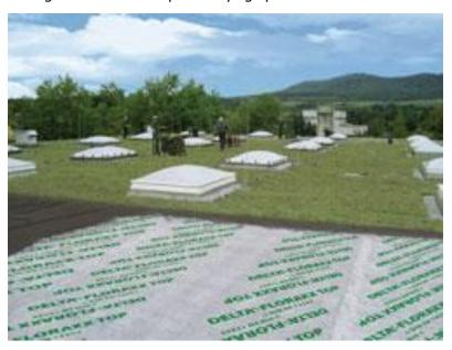
Ease and speed of installation is a huge benefit with both of these products, the sheet size of  $20m \times 2m$  for Delta-FLORAXX, while the FLORAXX Top option is supplied in  $10m \times 2.1m$  sheets (the extra 100mm geotextile width allows for overlap).
