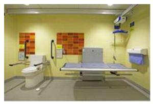
The height adjustability enables users to set the equipment to their convenience. The Clos-o-Mat toilet, with its integrated douching and drying facility, means the need for a carer to wipe the user clean after using the toilet is removed. It, and the changing bench, ensure optimum cleanliness and hygiene is achieved.
