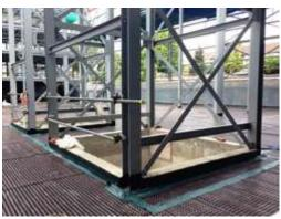
Delta MS500 was fixed to the walls with self-sealing plugs, and MS20 was applied to the floor and sealed to the wall membrane/upstands.
