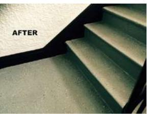
Work commenced with grinders and planing equipment to remove all existing floor coatings to the landing areas, treads, risers and upstands. Once all the floor coatings had been removed, operatives dealt with areas of cracking and spalling to the concrete substrate.
