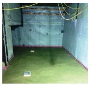
Delta cavity drain membranes work on the principle of allowing water to continue to penetrate the structure but control it in the air gap and divert it to a suitable drainage point or pump. A cavity membrane does not allow pressure to build up against the internal construction, and the air gap behind the membrane allows the structure to 'breathe' and dry out. The membranes are impermeable to water, and gas and water vapour, thus protecting the basement internal space from dampness.
