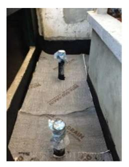
Cemplas operatives Installed Delta Duexan 2C including fillets at internal angles and fibre reinforcement. To the vertical area a 3mm rot proof protection board was applied, and the horizontal areas had a Delta Geo-Drain Quattro layer drainage sheet installed.
