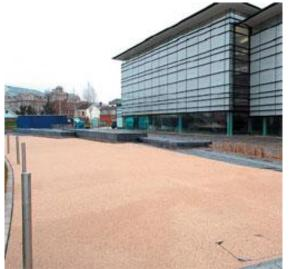
The **Resin Bonded**, and **Resin Bound** systems can also incorporate a waterproof membrane for use in suspended structures such as balconies and podium decks, and also **Resin Bound Tree Pit System** which is also decorative, but designed to be highly porous, allowing the tree to feed, and help to reduces the build up of litter and mess.
