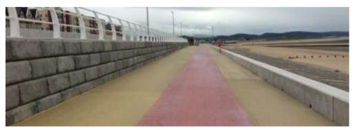
The flood defence is 470 metres in length and required standard protection designed for a 1 in 200 year storm with an allowance for 50 years of climate change.
