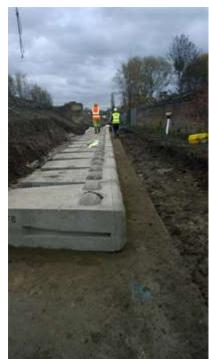
Around 175,000m³ of earth was removed during the extensive construction programme and Balfour Beatty decided to use CPM's Redi-Rock™ modular retaining blocks. Benefits of this product include offering a pleasing aesthetic look to the project, being fast to install and being delivered ready to use in any weather.
