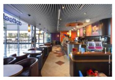
Providing excellent sound absorption where the soffit needs to be exposed to optimise thermal mass, their vertical linear aesthetic delivers a directional comparison to continuous suspended ceilings and enhances contemporary design trends.
