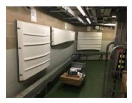
The third solution was to deploy simple flood gates that are manually closed across the corridors (and flood barriers across the doors) upon receiving notice of a flood. To improve the warning times, alarms were installed at strategic locations around the car park and connected directly to the security guard's office.
