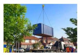
However, there was also no space around the building and only limited room to the rear. The team at AV Danzer were not fazed and brought in a 100-tonne crane to lift the unit over the shop and slot it in the space behind, which was just wide enough to allow the unit to fit and open the doors!
