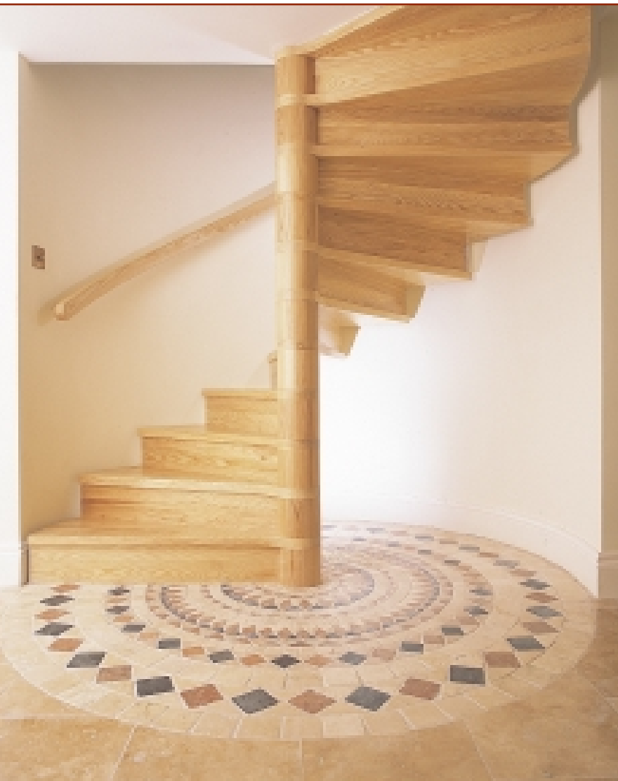
An American White Ash spiral built into a curved wall with smooth centre column and closed risers. The timber handrail is hung off the wall.
