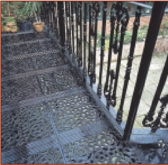
Cast aluminium plates 650 x 600mm or 1200 x 600mm with approximately 50% light through put.
