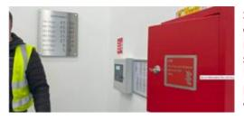
Safety Letterbox's contribution to this ambitious project comes in the form of their Secure Information Box (SIB), rigorously tested and certified to meet the stringent security standards of STS205 Resistance class BR2. Designed for both internal and external use, the SIB provides a reliable and secure solution for the storage and dissemination of important information.
